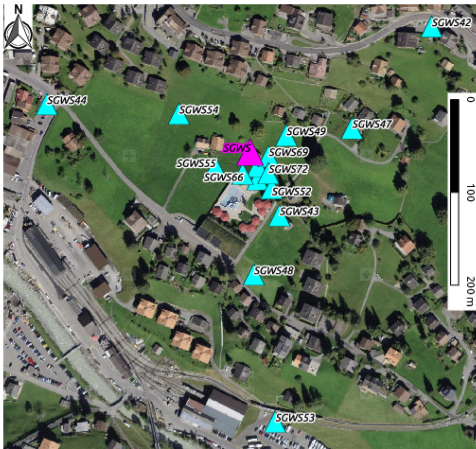
Figure 2: Aerial image of the survey site at Grindelwald with the strong motion station location and array configuration. Source of the aerial map: Federal Office of Topography.
