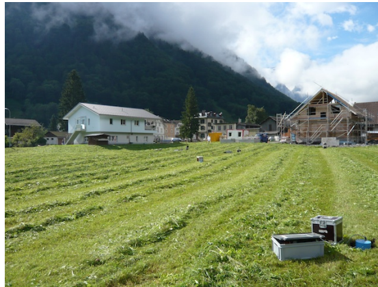
Figure 1: Picture of the site.
