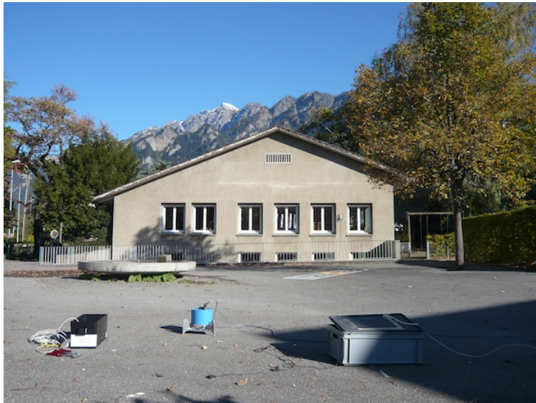
Figure 1: Picture of the site.
