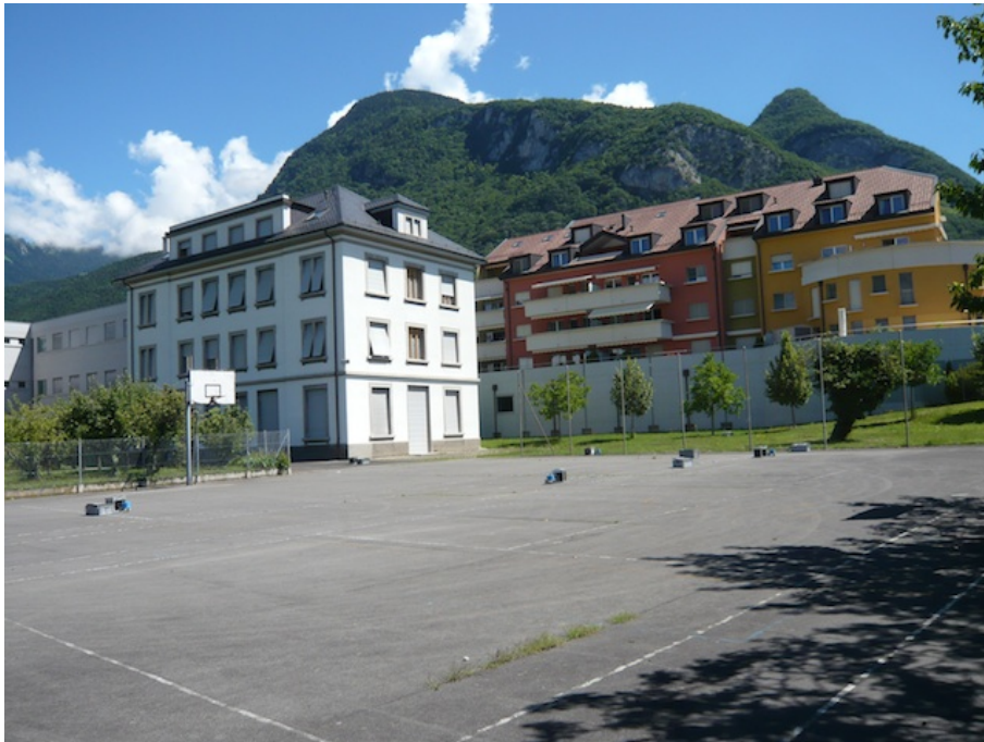
Figure 1: Picture of the site.
