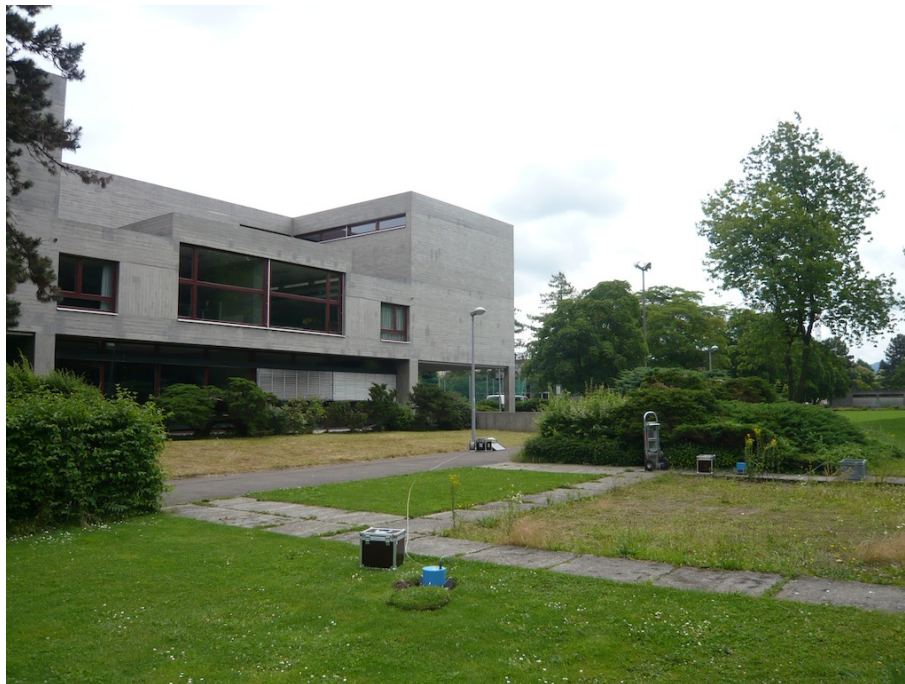
Figure 1: Picture of the site.
